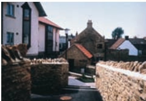
The Guinness Trust and Knightstone Housing Association have combined in Frome, Somerset, to create 'The Piggeries' – a mix of high density housing that responds sensitively to local context
